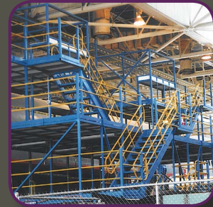
Custom designed access platform
